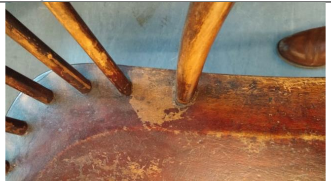
d. Water damage and wedge repair (left arm support)
